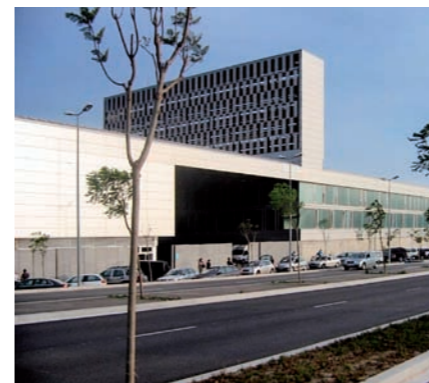
As perspiring athletes shower at the Joan Gamper Sports Centre in Barcelona, they also make sure that the environment stays clean: with hot water from solar energy thanks to SAUTER.
